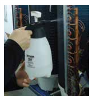
Corrosion Inhibiting coating inside the unit
